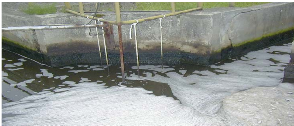
Figure 2. The exposure point – outlet stream on Plant II.
